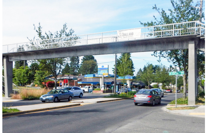
Existing conditions at Holman Rd NW and 13th Ave NW intersection
