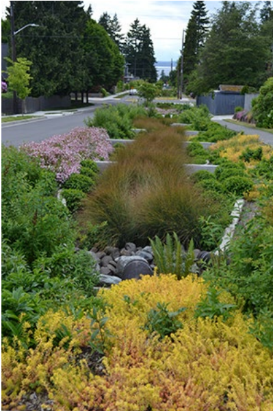
Green stormwater infrastructure uses special soils and plants to capture rainwater, clean it, slow it down, and soak it into the ground.
